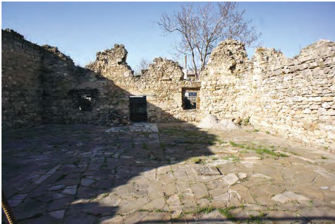
Fig. 2 – Sultan Kalavun Mosque (1287), walls and interior with remaining traces of the springer for the arches
